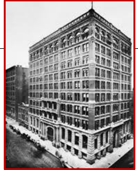
William Le Baron Jenney built the ten story Home Insurance Company building in Chicago (pictured above) which was the first true American skyscraper. Public Domain.
