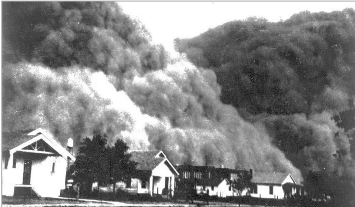
Photograph of dust cloud enveloping neighborhood, 1933
